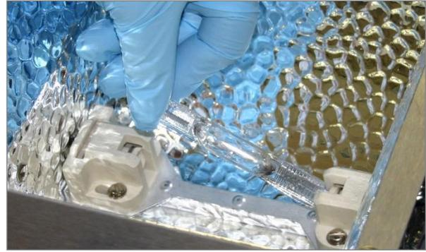
Step 6. Install the new bulb by following Steps 4 & 5 in the reverse order.
